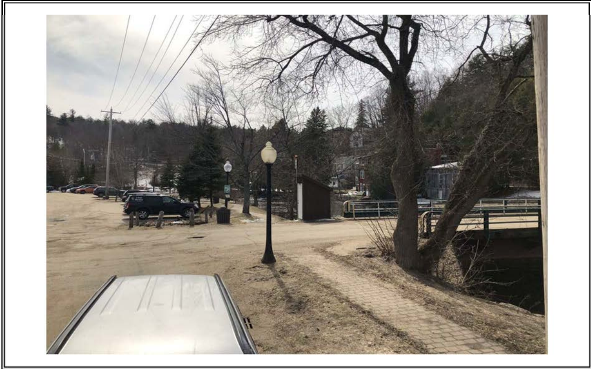
Photo No. 1 Alt. 2 - Looking south, existing Riverwalk and Dorsey Street bridge
