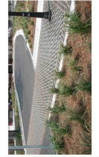
THERMOPLASTIC ASPHALT INLAY
