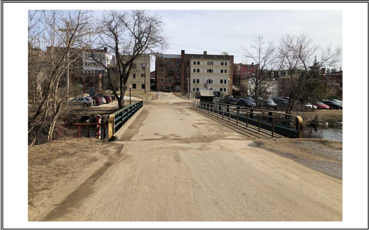
Photo No. 2 Alt. 2 - Looking east, Dorsey Street bridge with existing sidewalk
