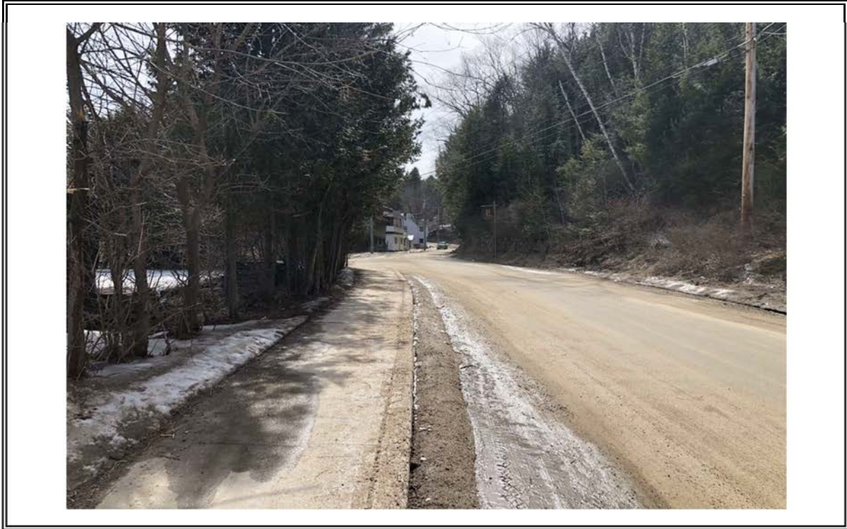
Photo No. 3 Alt. 2 - Looking south towards Dorsey Street bridge intersection
